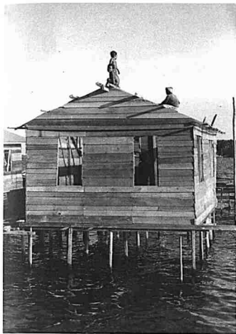
21 Village pile-house under construction.
